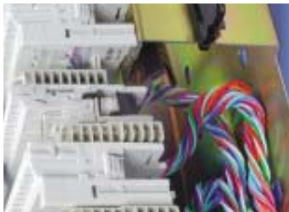
Permanent personal and equipment protection: no removing of the magazine for jumpering and testing
