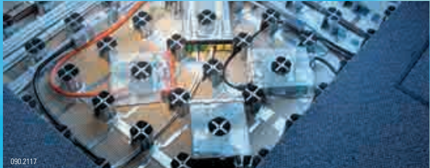
RCO Power in the stand floor: Base installation with round cables leads directly to the connection boxes; cable outlets supply the latter with power.
